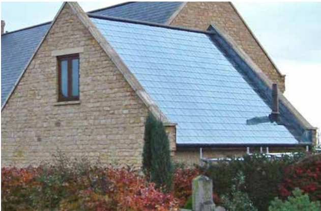
Figure 172: Positive example of implementing solar panels from the early design stage.
